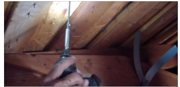
Fig 2b: Put a 2" screw through the roof deck.
