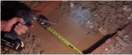
Fig 1: Insert screw to locate center of tube.
