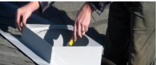
Fig 3: Use flashing as a template.
