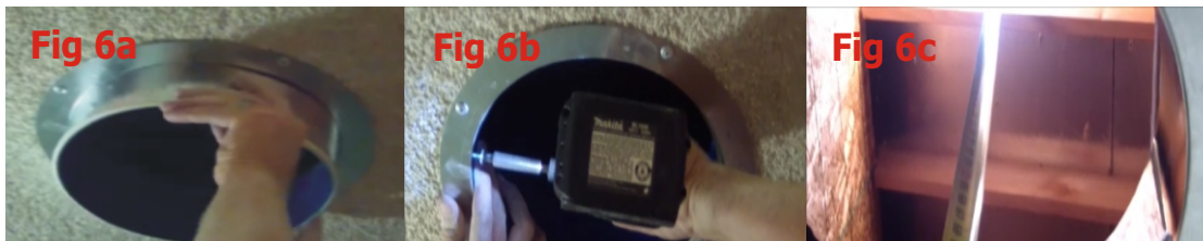
Slide in receiving collar, screw to fire ring, then measure tubing length.
